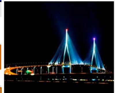
Incheon Bridge (ARUP website)
